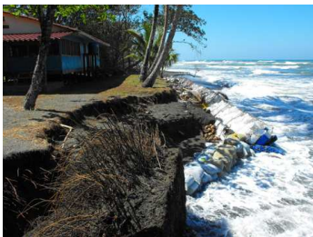
Figure 1. Extensive beach erosion at the South station.
